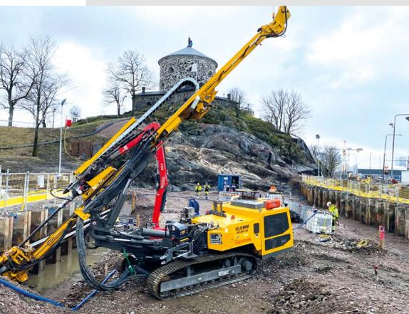
**Sweden** To secure a sheet pile wall with self-drilling anchors, our customer NCC in Gothenborg relied on a KLEMM KR 806-5G. **top**
