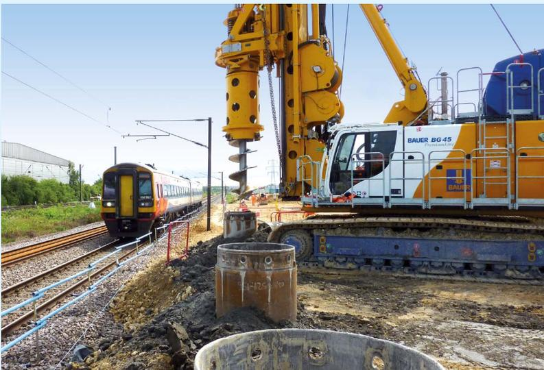
**United Kingdom** To increase traffic capacity between London and Edinburgh on the East Coast Main Line, the train route was expanded at Werrington. This project included the installation of piles in the immediate vicinity of the tracks, which required special measures to be taken to continue work without interrupting train traffic. **top**
