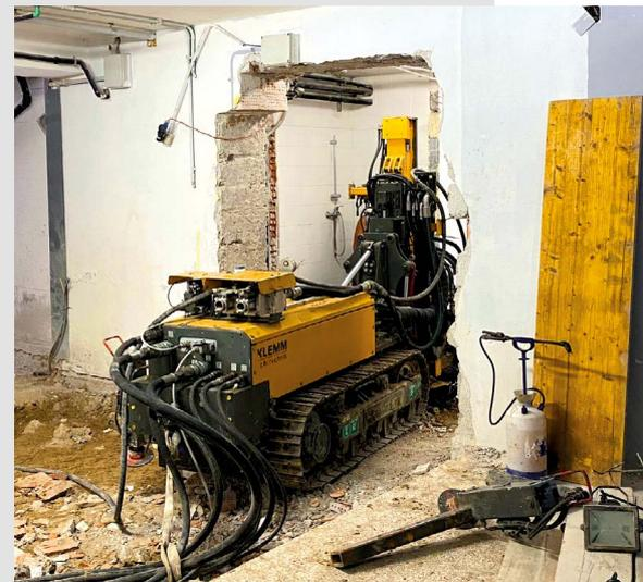
**Italy** Our customer Brenelli Costruzioni S.r.l. installed micropiles in the ground of a basement, using a KLEMM KR 702-2 and a KR 802-3S. **top**
