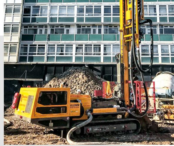
**United Kingdom** In London, Southern Piling UK carried out a micropile installation with hollow stem augers using a KLEMM KR 709-3G, up to a drilling depth of approx. 11 m. **top**
