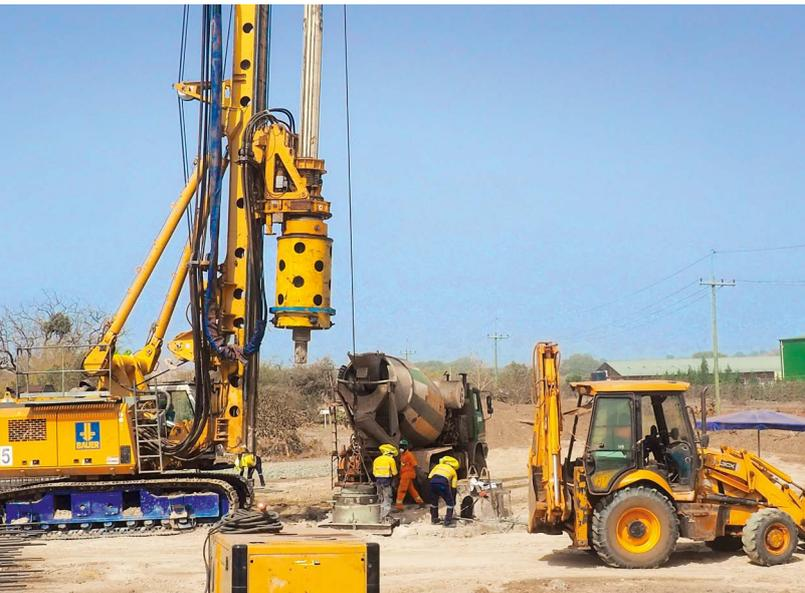
**Burkina Faso** A secant pile wall created using the Kelly drilling method up to a depth of 23 m forms the foundation for a new mine ventilation shaft. **top**
