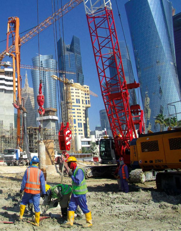
**Qatar** Using a BG 40 and a BG 28, a secant pile wall with a total of 112 piles was created for a pedestrian underpass in Doha. **left**
