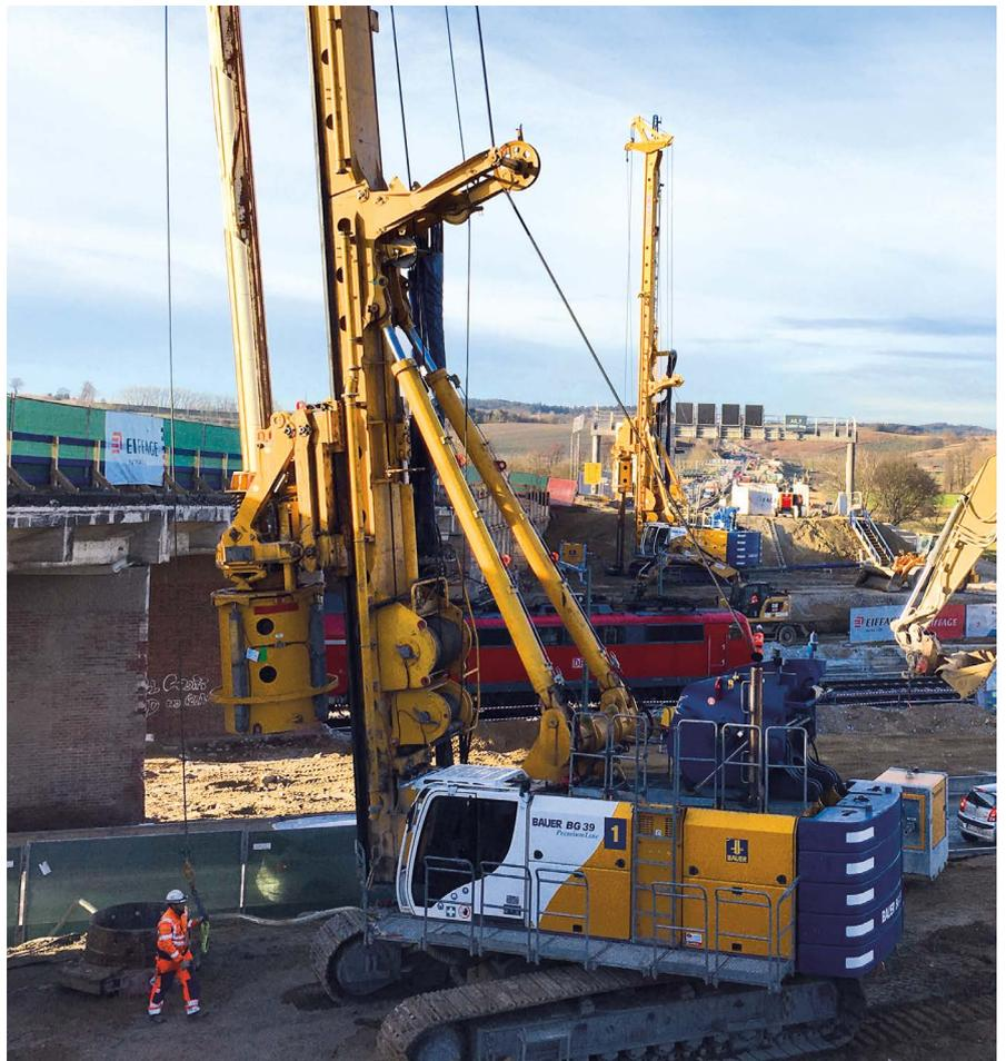
Using a BG 30, an excavation pit was created in **Mainz** for a residential building and hotel. First, 370 foundation piles were installed using the CFA method with drilling depths of up to 20 m, followed by retrofitting for the Kelly drilling method. **right**
