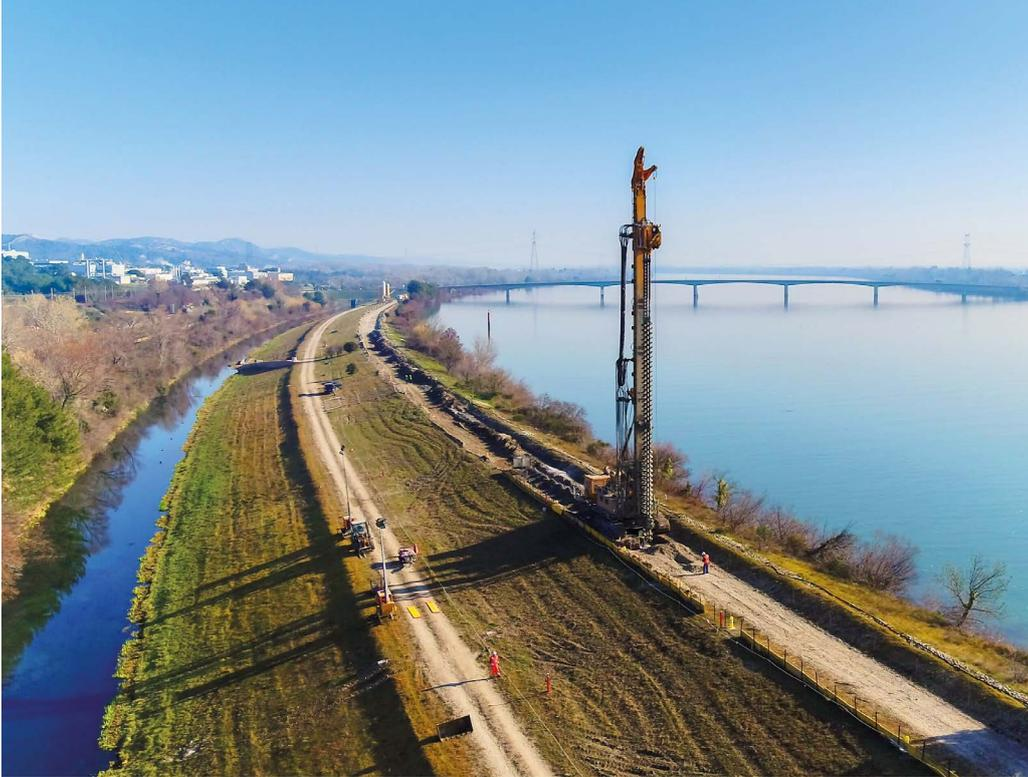
*A Mixed-in-Place wall was constructed for the remediation of a dike along the Rhone in Provence. The transport of construction materials was kept to a minimum thanks to the use of this method.*
