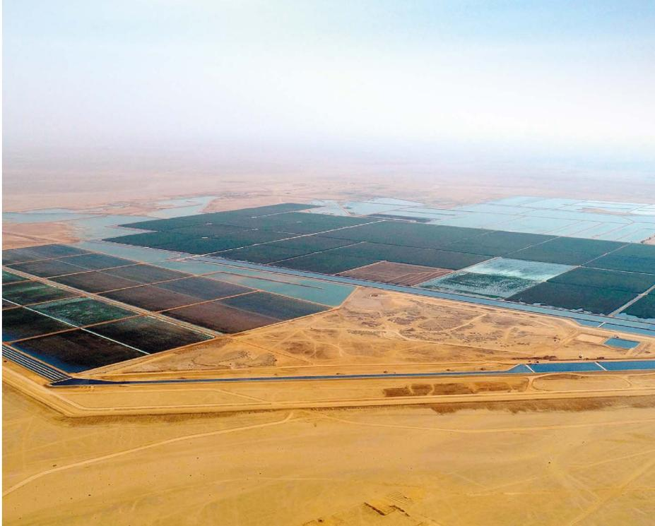
*After a third expansion, the reed bed treatment plant in Oman not only cleans 175,000 m<sup>3</sup> contaminated water daily, but the reduction in CO<sub>2</sub> emissions also meant that emission certificates for 114,000 t of CO<sub>2</sub> could be sold in 2019.*
