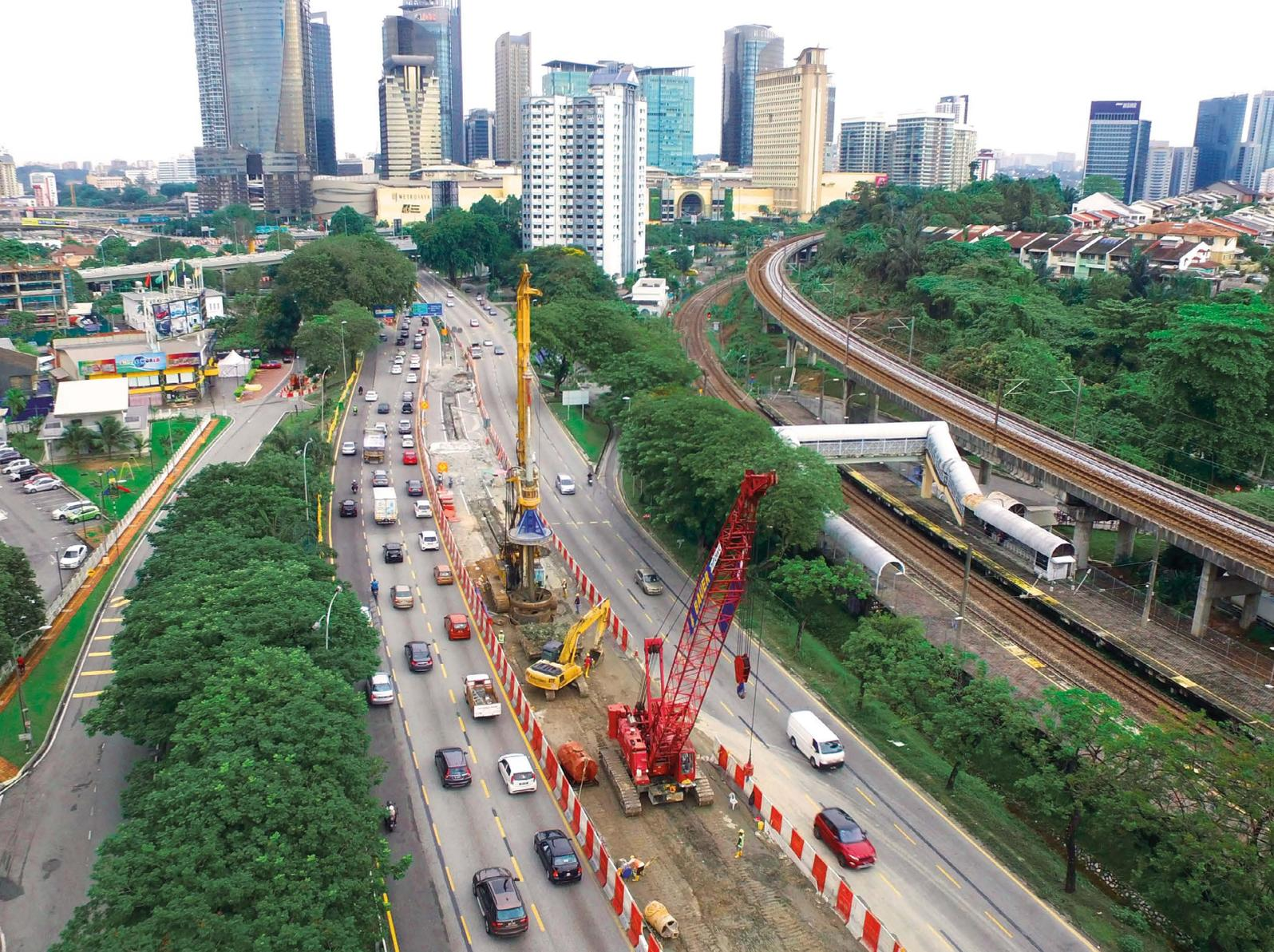
**Malaysia** For the new Setiawangsa-Pantai Expressway under construction to improve the traffic situation in Kuala Lumpur, 56 foundation piles were constructed using a BG 40 and BG 45. **top**
