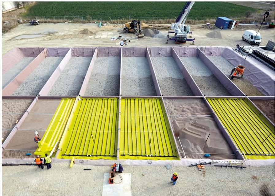
*A large-scale plant has been operating since 2014 based on the EcoVert® method to clean approx. 22 m<sup>3</sup> per hour of highly contaminated ground water from a former refinery location.*
