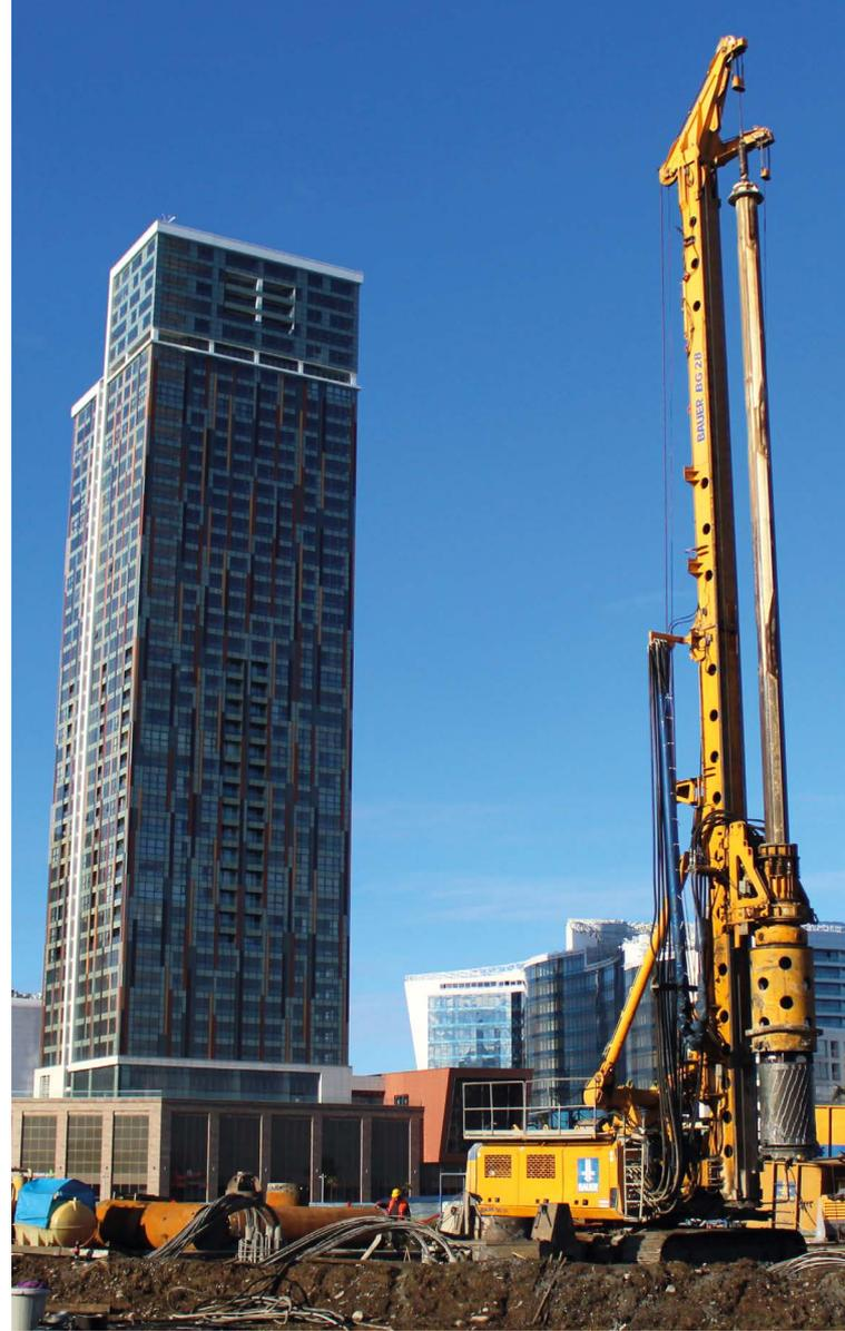
**Bulgaria** Good planning and organization was required for the execution of large-diameter bored piles for the Zhelezniitsa Tunnel, which will be the longest tunnel in Bulgaria when it is completed. Piles with a diameter of 1,500 mm and 1,800 mm were installed up to a depth of 25 m. **top**
