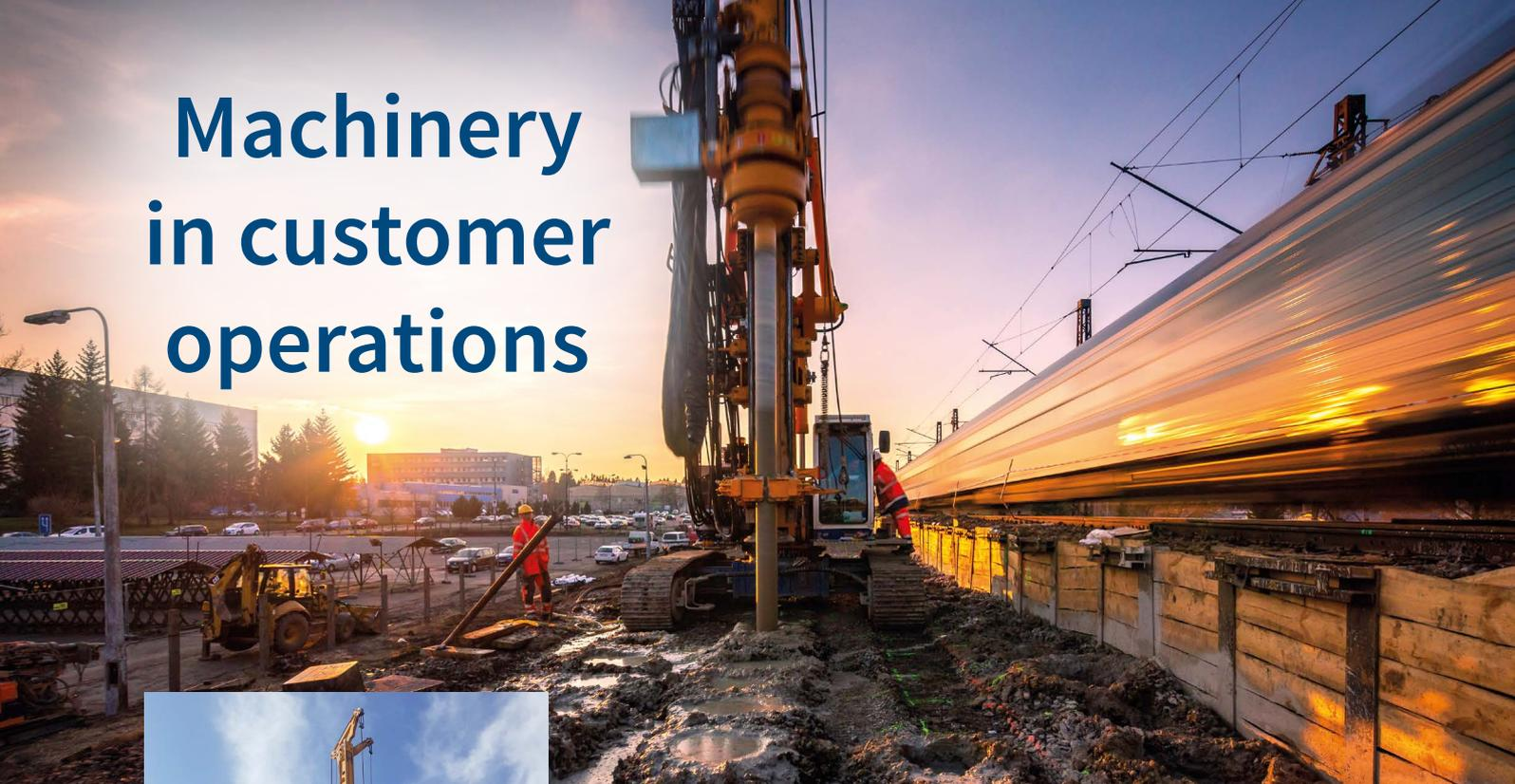
**Czech Republic** When carrying out ground improvements for a dual-track railway embankment, our customer Firesta-Fiser opted for a BG 20 H and the SCM method. **top**
