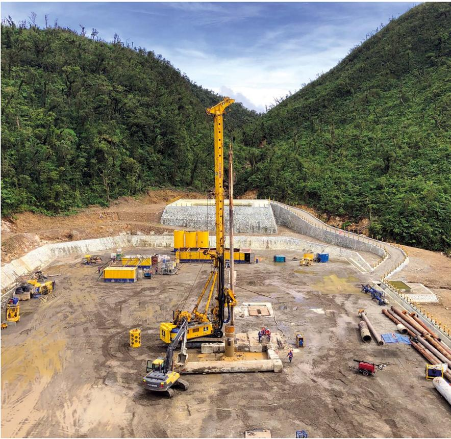
**Philippines** As part of a large investment program, drilling for a geothermal power plant was carried out on the island of Leyte. Over four months, multiple slurry stabilized drilling operations were carried out using a BG 40, up to a depth of 150 m. **left**
