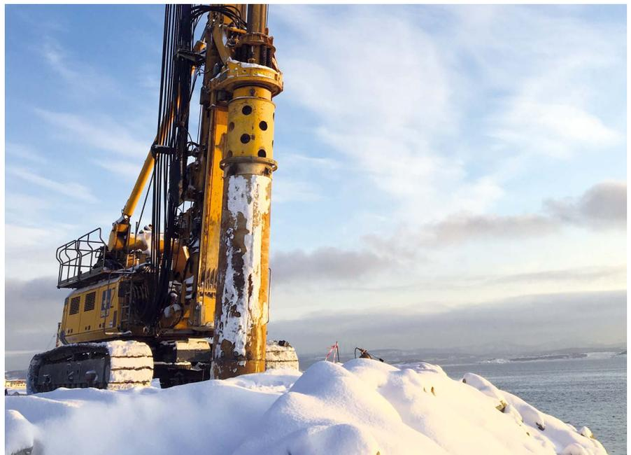
**Russia** For a new ocean engineering center in the Russian city of Murmansk, Bauer created a total of 2,540 lin.m. of piles with a length of up to 32 m. Construction was completed after 50 days of work. **top**
