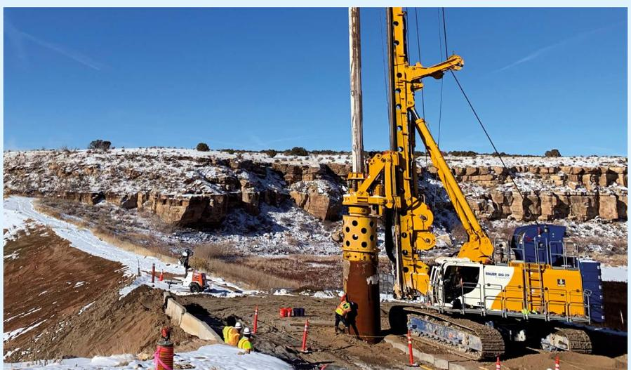
**USA** The Teller Dam is located within the U.S. army base Fort Carson near Colorado Springs. Bauer was contracted to seal the dam and will construct approx. 1,160 m<sup>2</sup> of secant pile wall as well as approx. 1,760 m<sup>2</sup> of grout curtains for this purpose. **top**
