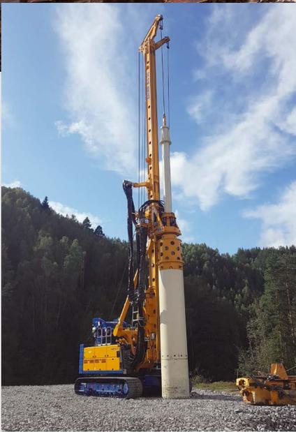
**Norway** The customer Keller Grundbau executed a bridge construction site with a BG 36 using the Kelly drilling method. **top**
