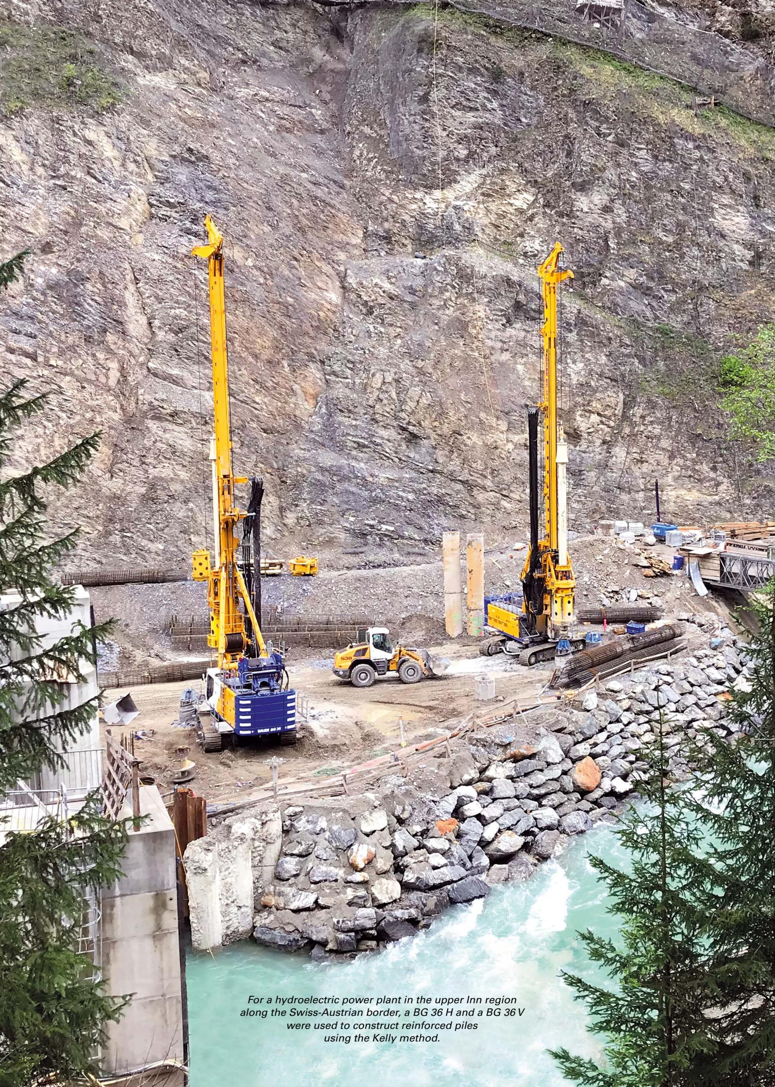
*For a hydroelectric power plant in the upper Inn region along the Swiss-Austrian border, a BG 36 H and a BG 36 V were used to construct reinforced piles using the Kelly method.*
