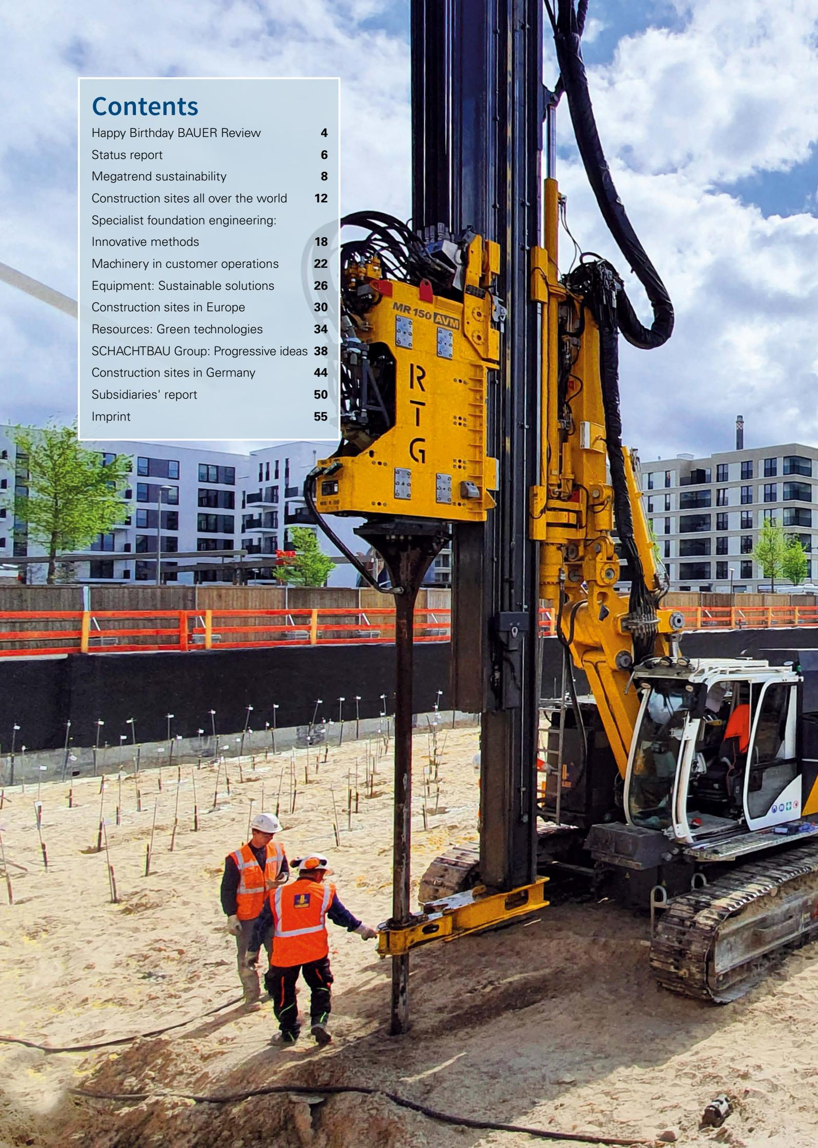
*An RTG RG 19T was used during work on the QHTrack project in Berlin. The excavation pit was horizontally sealed, using an environmentally compatible and sustainable LWS silicate gel base.*
