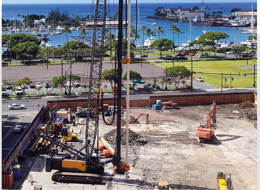
**USA** In order to reach a drilling depth of 44 m with the duty-cycle crane MC 128, we designed a special jib in collaboration with the company Berminghammer. After just two months, the MC 128 was used in Hawaii for the first time. **top**
