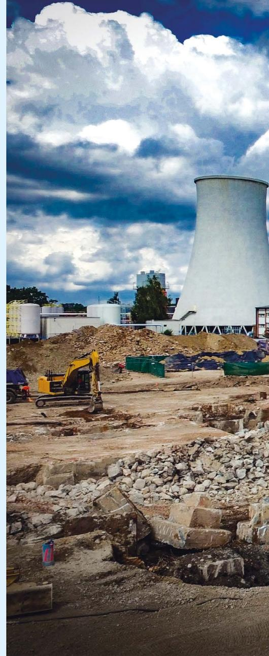
530 m long and up to 50 m wide: The excavation pit for the "QH Track" project in **Berlin** extends over an area of 16,000 m<sup>2</sup>. As part of the huge project "Quartier Heidestrasse" and in the immediate vicinity of the central station, a completely new district will be created here. For the encompassment of the excavation pit, approximately 23,000 m<sup>2</sup> of MIP wall was created along with a LWS base for horizontal sealing. **top**
