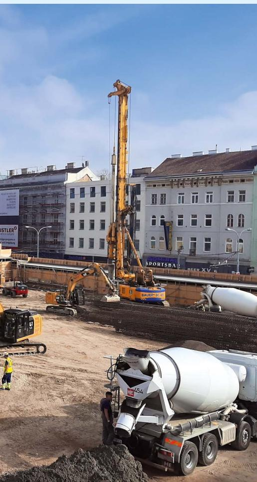
**Austria** A seven-floor IKEA furniture store is due to be built by 2021 at the Westbahnhof in Vienna. In a period of around eleven weeks, Bauer created around 5,100 lin.m. of in-situ concrete piles and around 5,400 lin.m. of drillings for the king pile wall. The deepest drillings went down to a depth of 36 m. **left**
