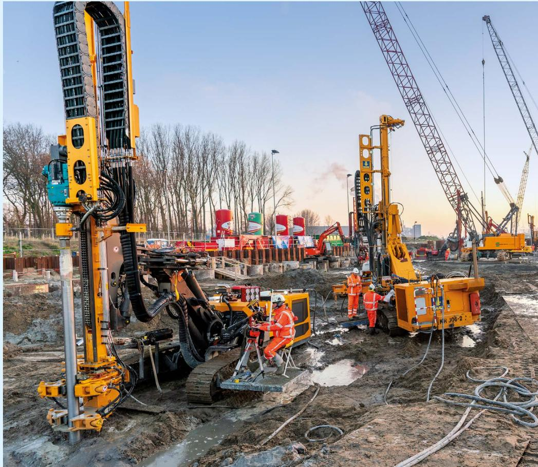
**Netherlands** For a new motorway link in Rotterdam, around 10,000 t of material were installed in the second-largest city in the Netherlands. A total of 4,500 GEWI® thread bar piles, that is, micro piles with threads, were required for the "Blankenburg connection" and executed by a total of eleven teams using eleven KLEMM KR 806 rigs. **top**
