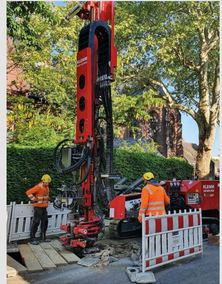
**Germany** GbE Grundbau Essen GmbH successfully carried out fill drilling and exploratory drilling in Bochum, using a KLEMM KR 801-3GS. **top**
