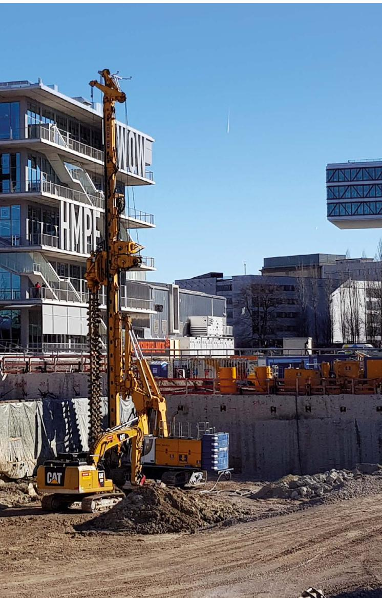
Near the Ostbahnhof station in **Munich** on the former premises of the Optimol company, a new office building will be constructed as a high-rise with three underground floors. For the execution of the excavation pit, a total of approx. 7,400 m<sup>2</sup> MIP retaining structures were constructed and secured with 330 anchors in one to two layers. In addition, foundation piles were constructed up to a drilling depth of 29 m. **left**
