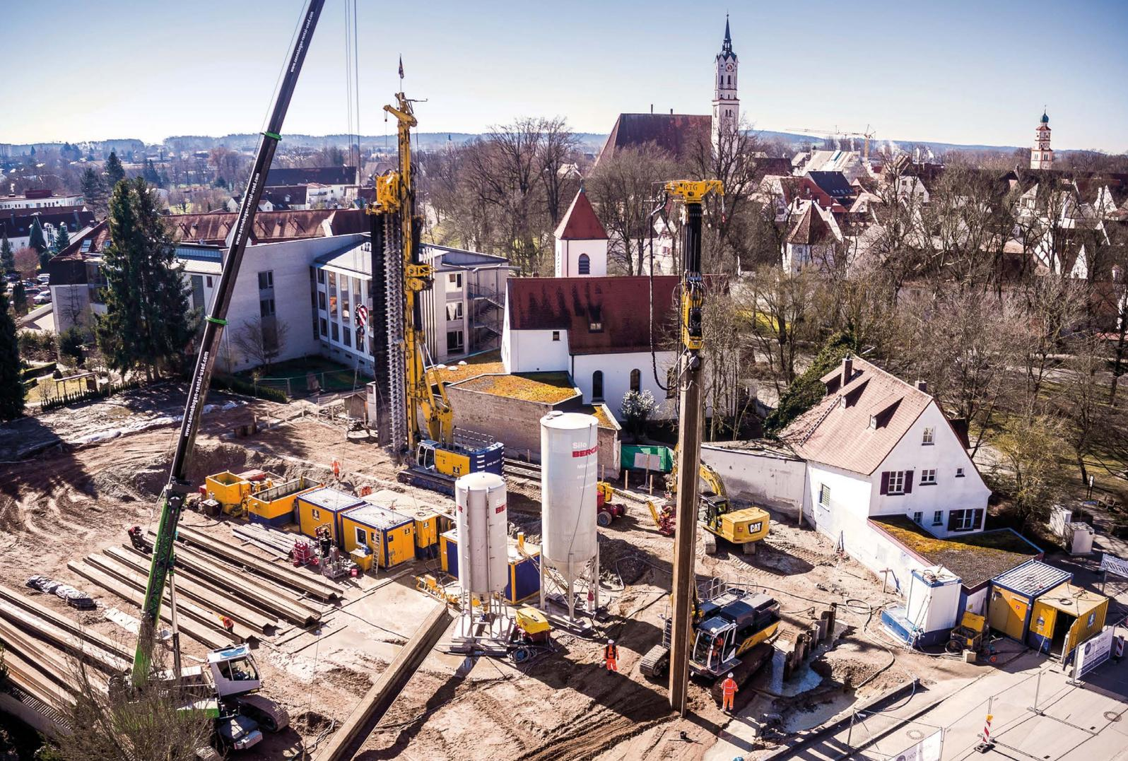
In **Schrobenhausen**, the home-town of Bauer, a new residential complex with two houses and a total of 2,400 m<sup>2</sup> living space will be created by 2021. To seal against ground water, the excavation pit was made impermeable before excavation with a retaining wall using a combination of sheet pile wall construction and the Mixed-in-Place method. **top**
