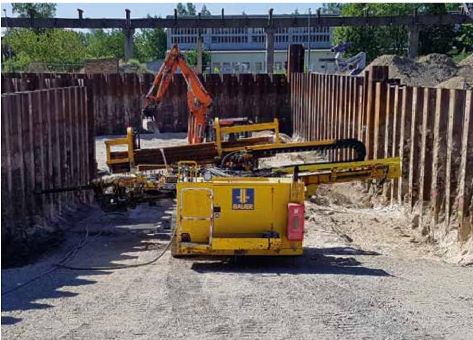
To remediate the contaminated site at the **Schwarze Pumpe** industrial park, all specialist foundation engineering and soil replacement measures are being implemented jointly by Bauer Resources and Bauer Spezialtiefbau. For soil support, approx. 1.3 km of sheet pile walls are being fitted and a further 147 individual sheet pile wall boxes are to be built over the course of the works for excavation of over 286,000 t of soil. **Left**
