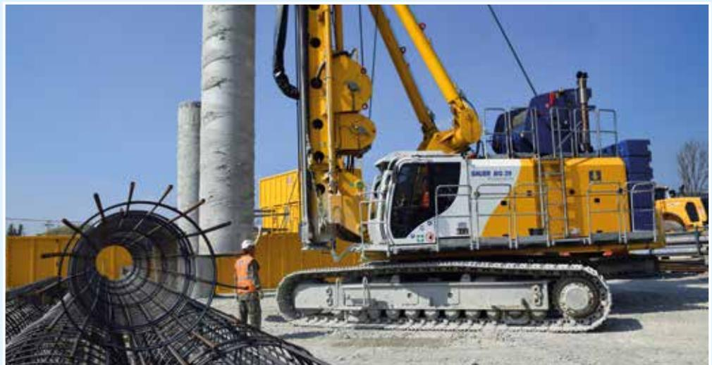
To sustainably alleviate congestion caused by truck traffic in downtown **Rosenheim**, a bypass road called the Rosenheim Westtangente (west bypass) is being built. To build the new major bridge, approx. 15,000 m vertical drains and 253 large-diameter bored piles are required in Rosenheim marine clay, an extremely sensitive soil stratum with low load-bearing capacity and a high water content. **Top**
