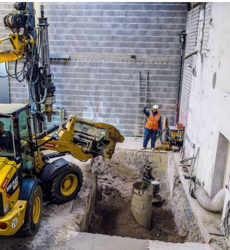
*Bauer Umwelt's environmental technologies help clean sites where water and soil have been polluted by industry. Replacement boring was carried out for a customer in Wuppertal under extremely cramped conditions.*
