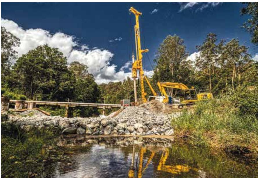
**Australia** To build the pillar foundations for five bridges in Queensland, two BG 30 drilling rigs were mobilized just two weeks after the contract was awarded. For each bridge, two abutments with four piles were driven up to 3.5 m into the bedrock. **Top**
