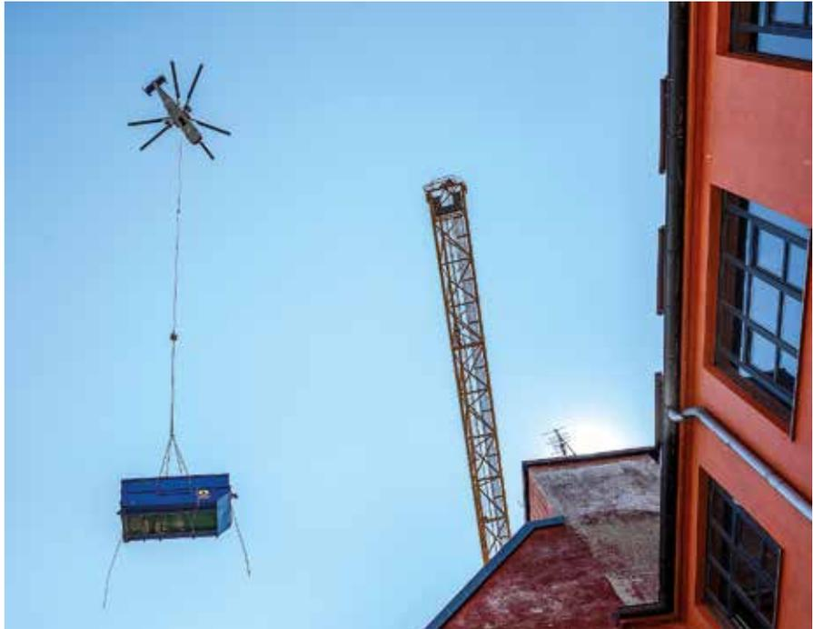
*This 4.5 t water purification system from Bauer Umwelt was lifted by helicopter from an excavation pit in downtown Munich.*
