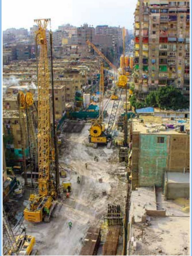
**Egypt** Bauer has been involved in expanding the metro in Cairo for several years. The specialist foundation engineering works for phase 3 of the mega-project are currently underway. The works for four of the six subway stations and two of the seven ventilation shafts have already been successfully completed. In total, approx. 250,000 m<sup>2</sup> of diaphragm wall are being built. **Top**
