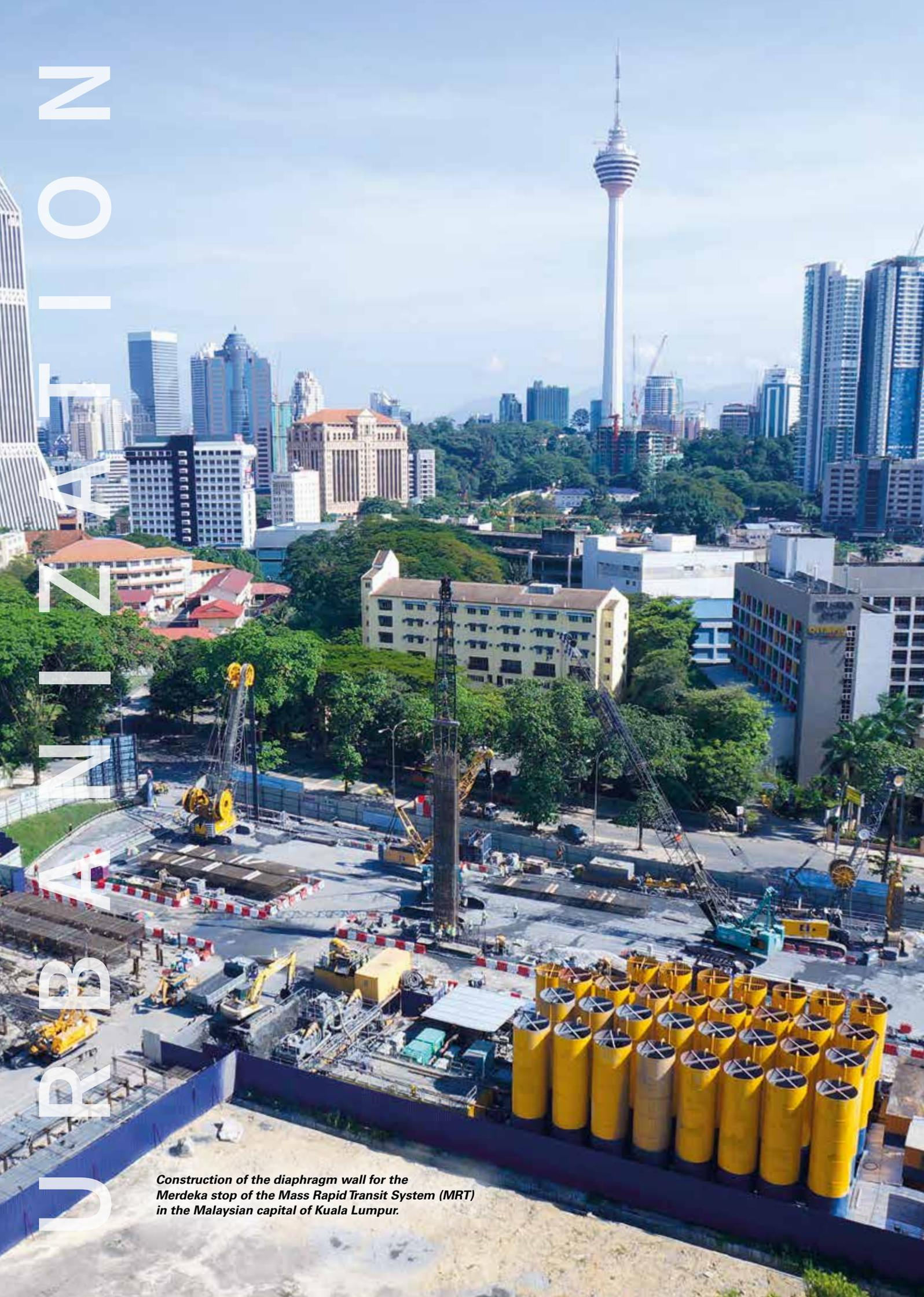
*Construction of the diaphragm wall for the Merdeka stop of the Mass Rapid Transit System (MRT) in the Malaysian capital of Kuala Lumpur.*
