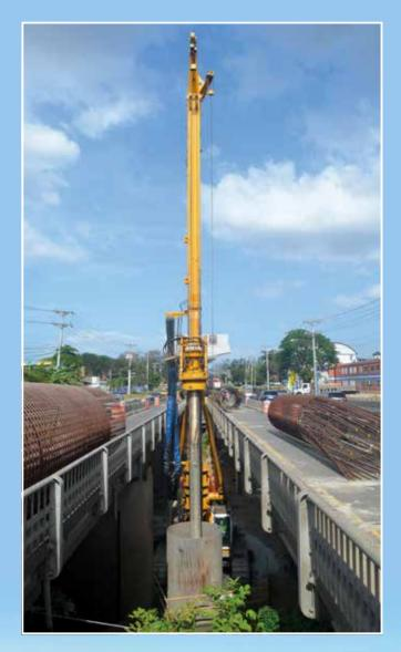
**Panama** From January 2016 to March 2018, a BG 28, BG 39 and BG 40 were used to install 783 bored piles up to 2,250 mm in diameter to depths of up to 43 m for the foundation of the continuous elevated metro line 2 in Panama City. **Left**
