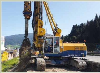
**Austria** On the A10 Tauern motorway south of Salzburg, noise barriers are being built on a foundation consisting of 9,900 m of bored piles. Two BG 20 H and BG 15 drilling rigs are being used. **Above**
