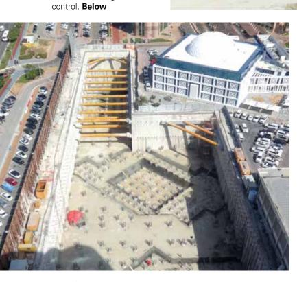
**Dubai** A gigantic shopping center is being built as part of the future Dubai II Big Box Retail Park. The excavation pit was constructed using secant and contiguous pile walls as well as soldier piles with wooden laggings over a length of 780 m. The project also included 1,754 foundation piles and 200,000 m<sup>3</sup> of excavation. **Right**
