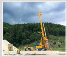
Estonia Our Baltpile customer OUe used three BG 30, BG 36 V und BG 40 V specialist foundation engineering rigs and a KR 806 anchor drilling rig to construct the excavation pit for a multifunctional building complex in the Tallinn yacht harbor.
