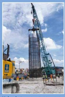
**Malaysia** Bauer installed bored piles with diameters of 1,350 to 3,500 mm in hard rock for an inner-city motorway bridge in Kuala Lumpur. The contract also included a test program consisting of a group of six test piles. **Above**
