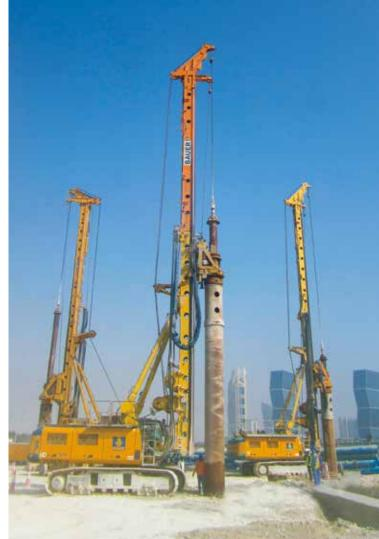
**Qatar** Three BG 28 and one BG 40 were used to install 999 piles for the foundation of giant rice silos on a 5,000 square-meter site at the port of Hamad, south of the capital Doha. **Right**
