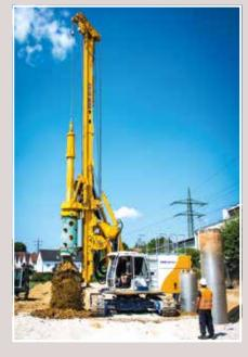
Austria Vienna-based Porr Bau GmbH uses a BG 45 in Kelly drilling mode to construct a bridge foundation that is 24 m deep and 1,500 mm in diameter for a town bypass in Oberau, Bavaria.
