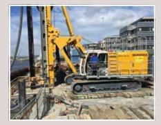
**Sweden** Our customer Skanska Sverige AB uses an RM 20 pile driver with the air hammer drilling method to drive piles measuring 406 mm in diameter to a depth of 60 to 110 m for the foundation of the new Goeta Aelvbron bridge in Gothenburg.
