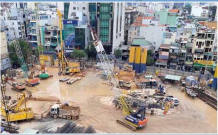
**Philippines** Sixty-five 2.8 m diameter bored piles were installed on land and seventy-four 3.4 m diameter offshore piles were installed in the San Juan Riverbed for the extension of the Metro Manila Skyway. The maximum depth of the piles is 44 m. **Below**
