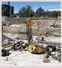
China Shenzhen Shenglong Construction Co. Ltd. uses a BCS 40 cutter to build Niuhu Station on Shenzhen Metro Line 4.
