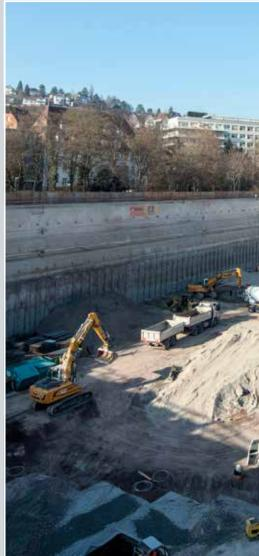
From November 2017 to March 2018, Bauer constructed around 7,200 m<sup>2</sup> of MIP wall with a record depth of up to 23.8 m for a hotel and residential construction project in the Rebstock district of **Frankfurt** am Main. The project also included 1,300 meters of anchors meters, 20,000 m<sup>3</sup> of excavation as well as groundwater control.
