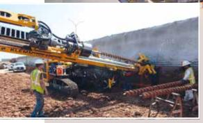
**USA** Our customer Earth Reinforcement used a Klemm KR 806-3G anchor drilling rig to install thousands of anchors to reinforce Sam Houston Lane in Pasadena, Texas. **USA** Our customer Malcolm Drilling used a CBC 25 cutter and a MAT BE 550 desander for slope stabilization below the Prado dam on the Santa Ana River in Corona, California for the construction of a concrete diaphragm wall.
