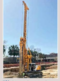
**USA** Schnabel Foundation Company in Texas uses a BG 20 H to install piles measuring 610 mm in diameter up to 9 m deep into the ground for an office building in San Antonio.
