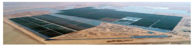
The plant-based purification facility in Oman not only cleans 175,000  $m^3$  contaminated water daily, but the reduction in CO<sub>2</sub>emissions also meant that emission certificates for 114,000 t of CO<sub>2</sub> could be sold in 2019.
